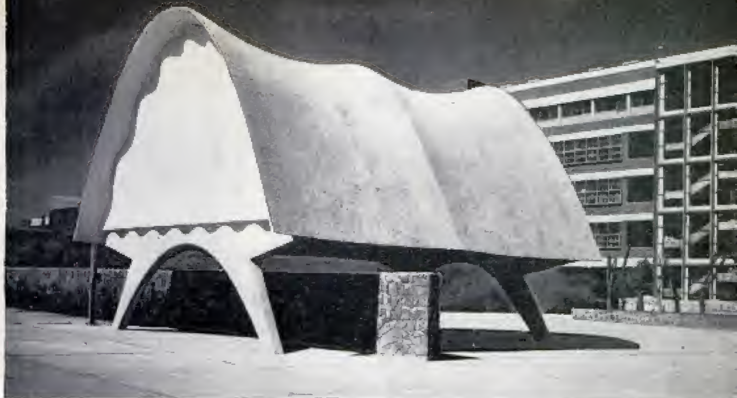
Mounted on stilts, the Pavilion of Cosmic Rays houses automatic neutron counters and ionization chambers
